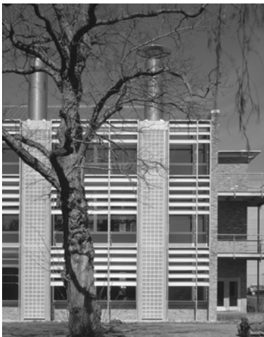
Figure 10.A.3. Solar chimneys in the Environmental Building, Building Research Establishment, Garston (UK).
