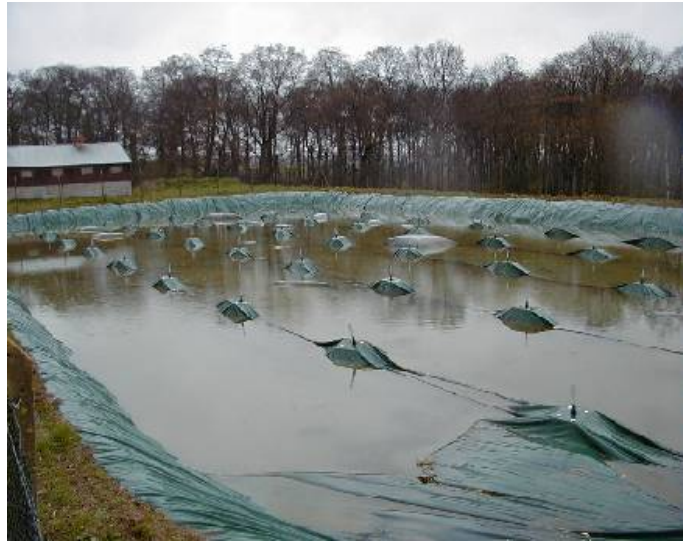
Floating tank/lagoon cover
